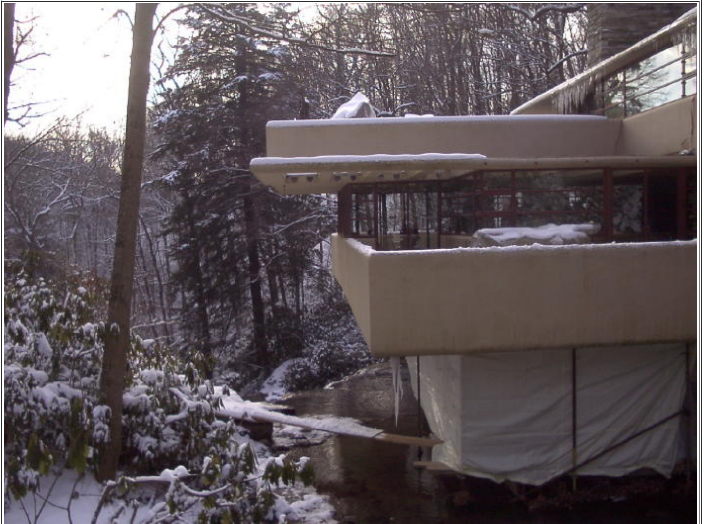
Looking downstream. The staircase was under construction, hence the wrapping.
